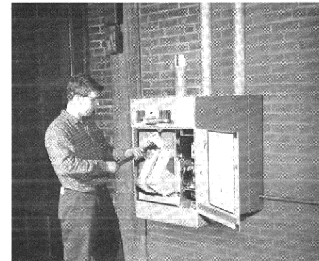
6 current limiting fuses being inserted in assembled starter.
