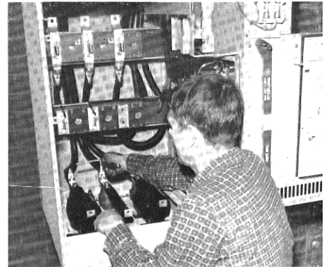
4 line and load cables connected to disconnect stabs and current transformers
