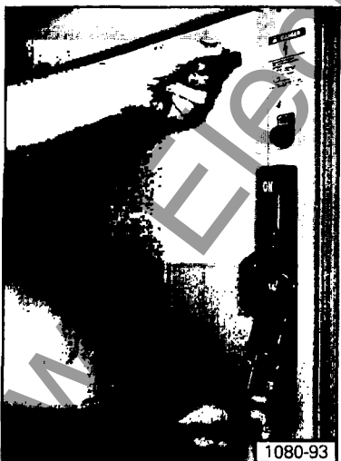
Figure 8. Procedure for defeating the door-handle interlock
