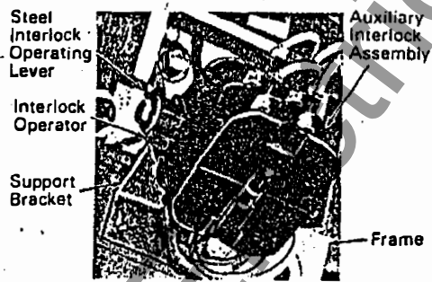
Fig.6 - Auxiliary Interlock Assembly
