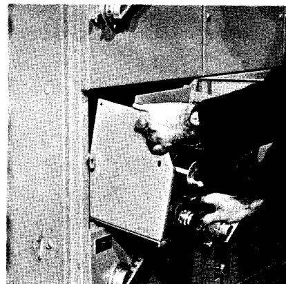
Fig. 13 Control Unit Withdrawal
