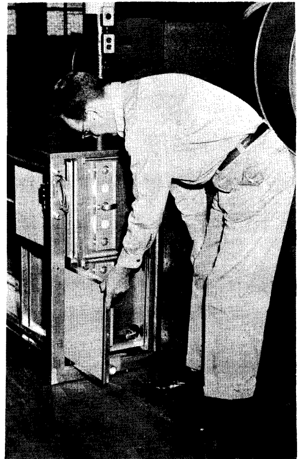
Figure 15. Installing After-Filters
