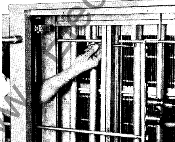
Fig. 13 Connections Between Ionizers
