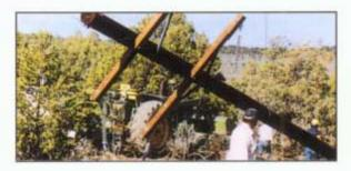
"Framing the pole on the ground offers significant construction savings with lightweight Hi\*Lile insulators."
