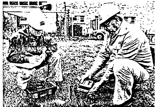
Measuring the resistance of a ground system on a pad-mounted transformer at a manufacturing plant.
