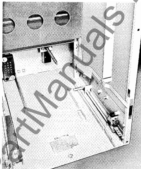
Fig. 22. Indoor and Outdoor: Close-up, Position Interlock (Locked)
