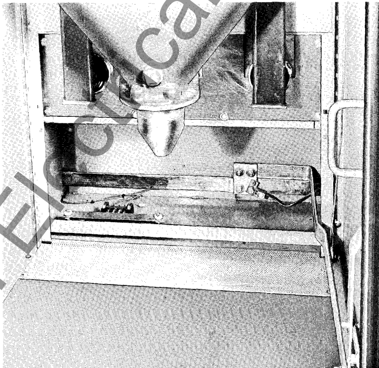
Fig. 12. Outdoor: Line Module with Rear Sheet Removed
