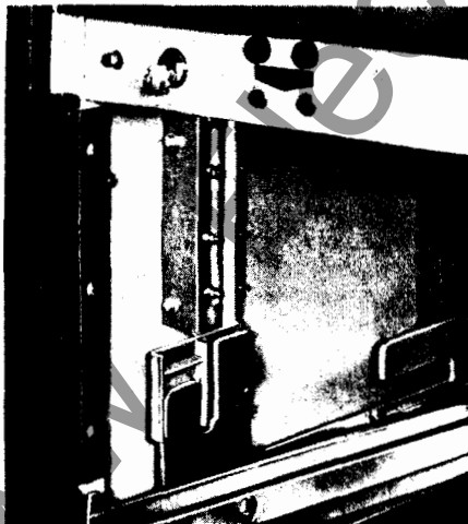
Figure 15: Key Interlock - Blocking Position
