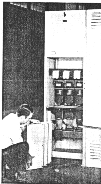
figure 13. Removing barriers of main bus compartment. Buses also accessible from breaker compartment.
