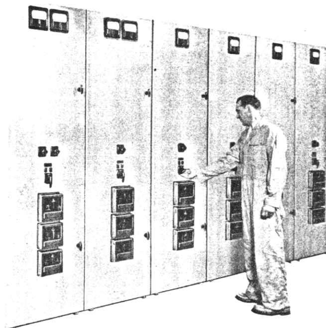
figure 5. Turning on power with control switch: Two metal barriers are between operating and breaker when circuit is energized, providing complete safety to operator.
