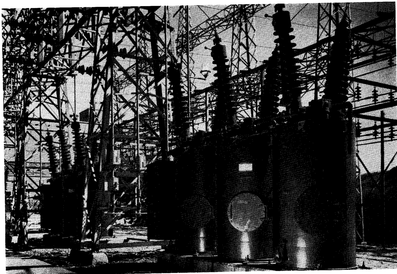
FIG. 14. Installation of Type GM Oil Circuit Breakers Showing Manholes for Inspection and Maintenance
