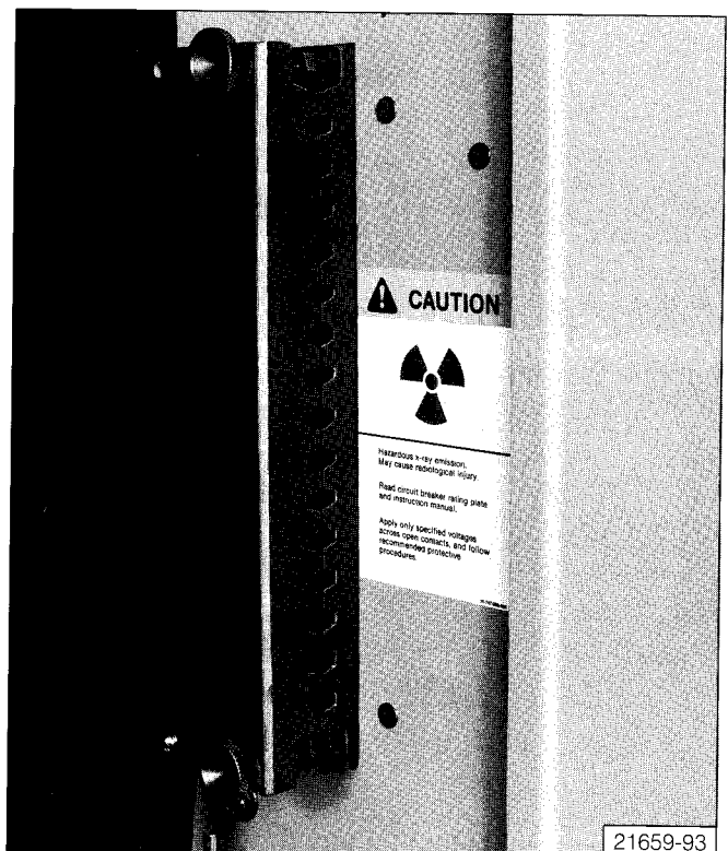
Figure 7: Split Plug Jumper Connected to Circuit Breaker.
