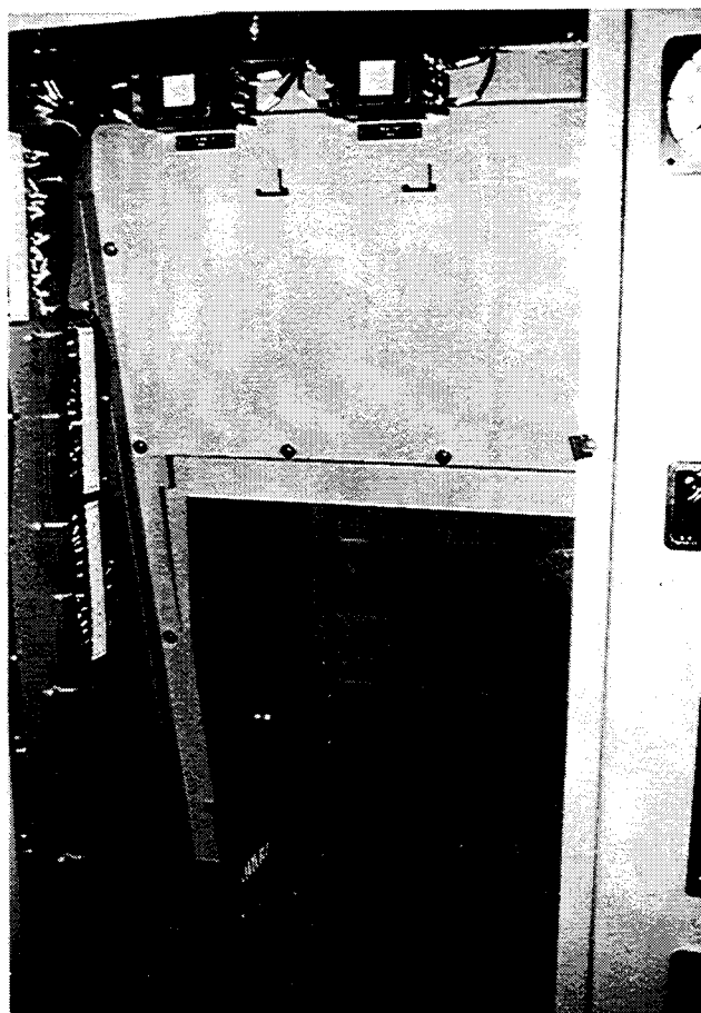
Figure 30 Cubicle Barrier for Type MSV Circuit Breaker
