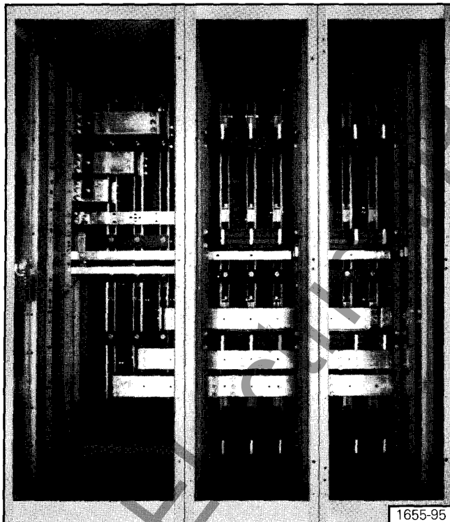
Figure 13. Typical Bus Bar Arrangement
