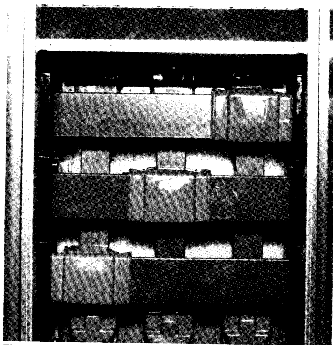
Figure 12c. Insulation Boots Installed. Unit is ready for reinstallation of main bus barrier (R, Figure 16a ).
