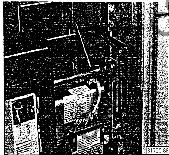
Figure 14. Key Interlock Located in Circuit Breaker Compartment.
