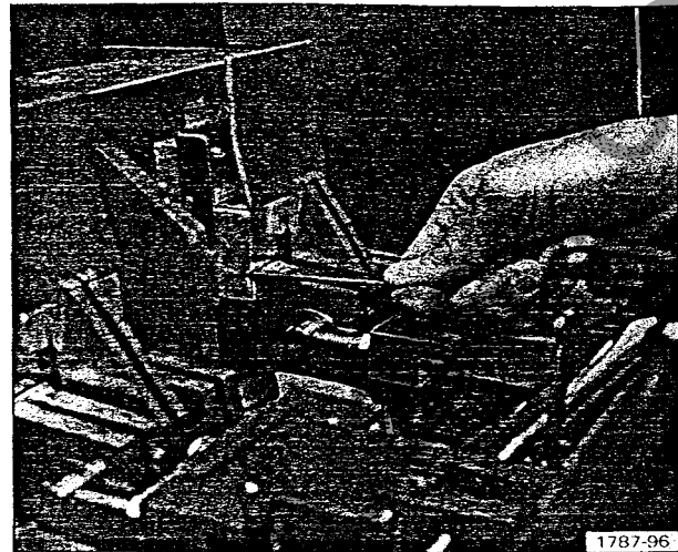
Figure 6a. Check of Main Contact Make (Compression) using GO/NO-GO Gauge
