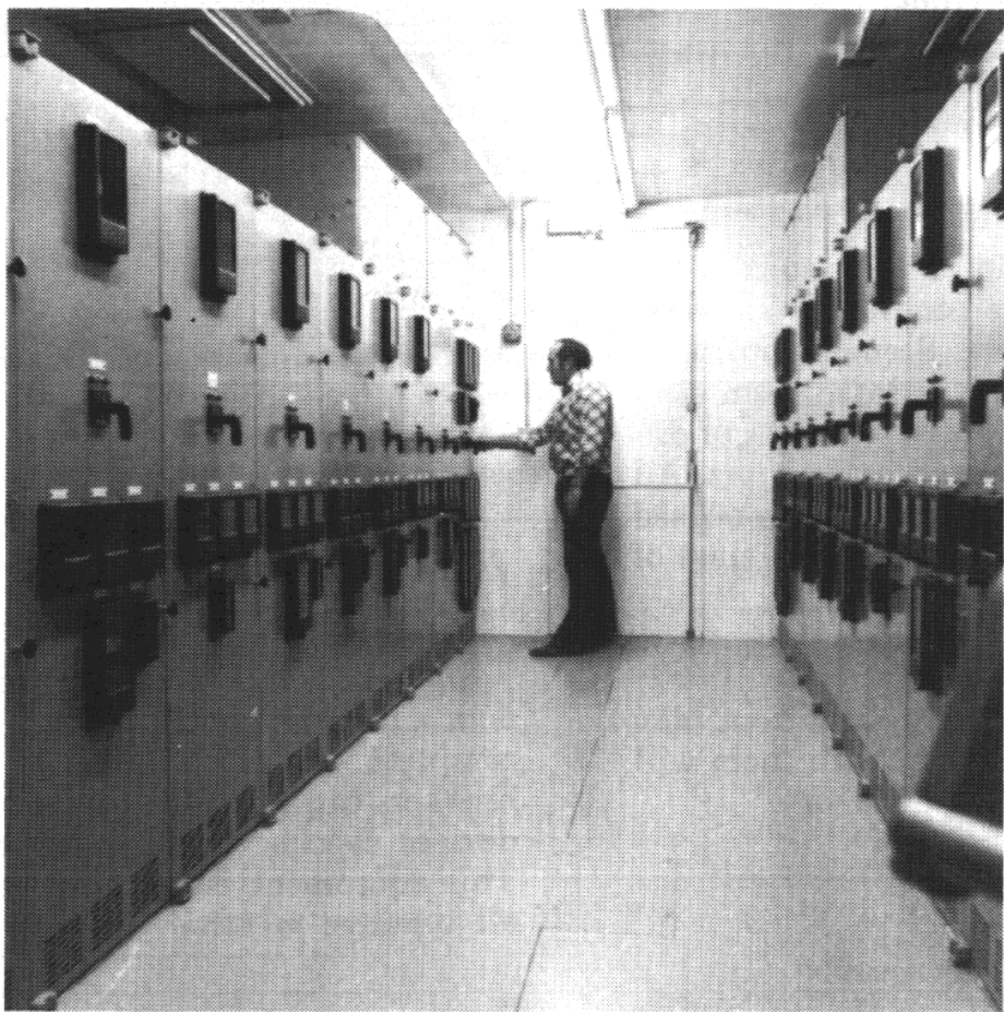
Figure 1. 5 KV Indoor Switchgear Installation
