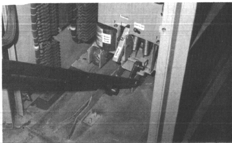
Figure 76. Racking Lever in Position to Move 5 kV Breaker to Fully Connected Position
