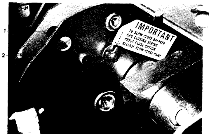
Fig. 11 Slow Close Pin On Flywheel
