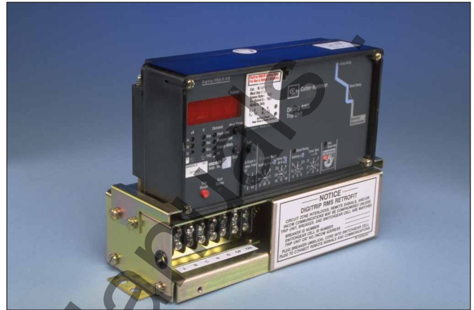
Fig. 3 Overview: Trip Unit mounted to the Aux. CT Module.
