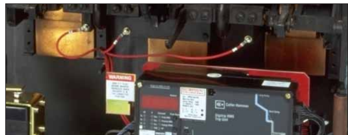
Fig. 18 PT Wires connected to the Phase Frames.
