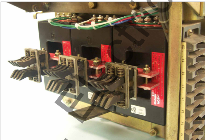
Fig. 8 Finger Clusters Reinstalled on the Bottom Breaker Studs.
