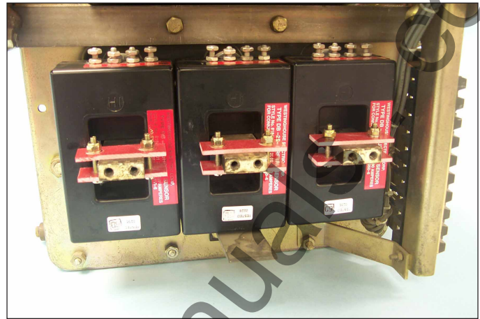
Fig. 5 Sensor Spacers Installed on the Bottom Breaker Studs.
