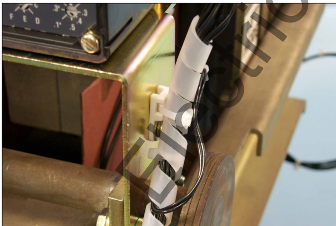
Fig. 58 External Harness Connected to the Trip Unit.
