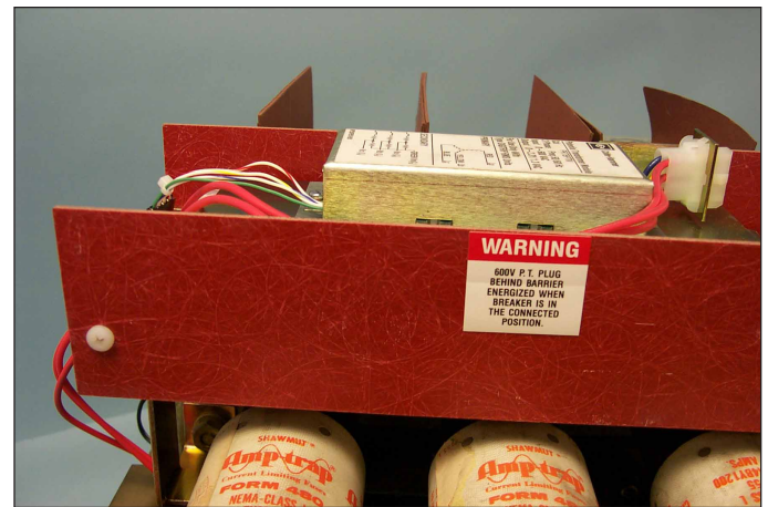
Fig. 26 PT Warning Label Installed on the Rear Aux. CT Module Insulation Barrier.
