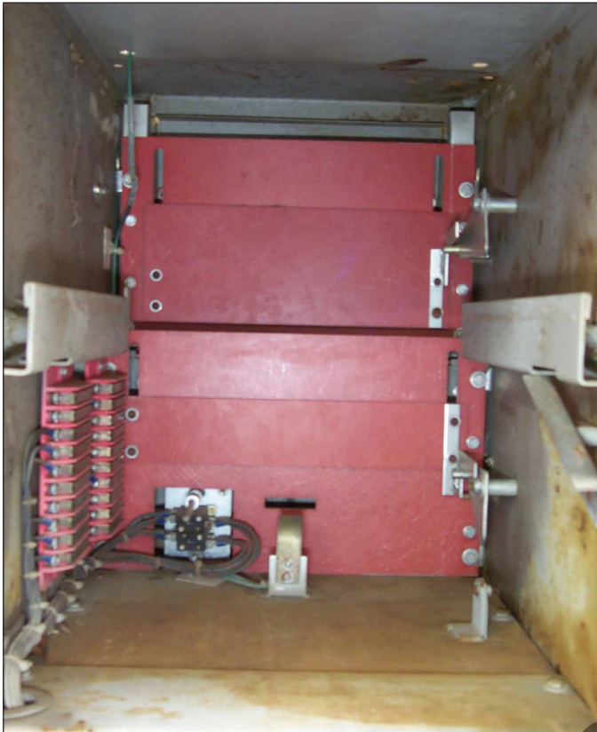
Fig. 62 The Inside of the Breaker Cell.
