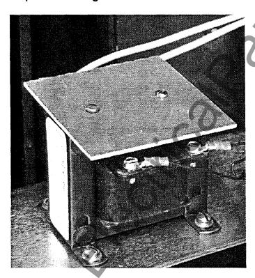
A. Align the holes in the Breaker Mounted CPT with the pre-drilled holes on the left side of the Trip Unit Mounting Platform. Secure the CPT to the Trip Unit Mounting Platform using the (4) .190-32 x .500" screws, (8) flat washers, (4) lock washers, and (4) nuts supplied. Note that the X1 and X2 terminals face the front of the Breaker.
