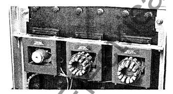
F. Reinstall the Finger Clusters and secure them using the original hardware.
