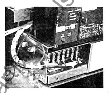
G. Route the DTA Extension Harness between the Glass Poly Insulation Barrier and the back of the Trip Unit, then down along the back edge of the right Trip Unit Support Bracket and into the Breaker to the DTA Assembly. Connect the wire from the DTA Extension Harness marked with "+" to the terminal to which the "+" DTA Wire is attached and the unmarked wire to the other terminal.
