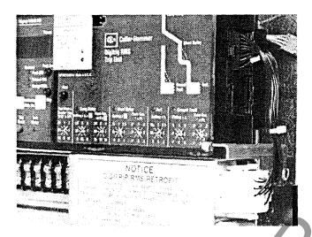
Step 5: Installing the Trip Unit
