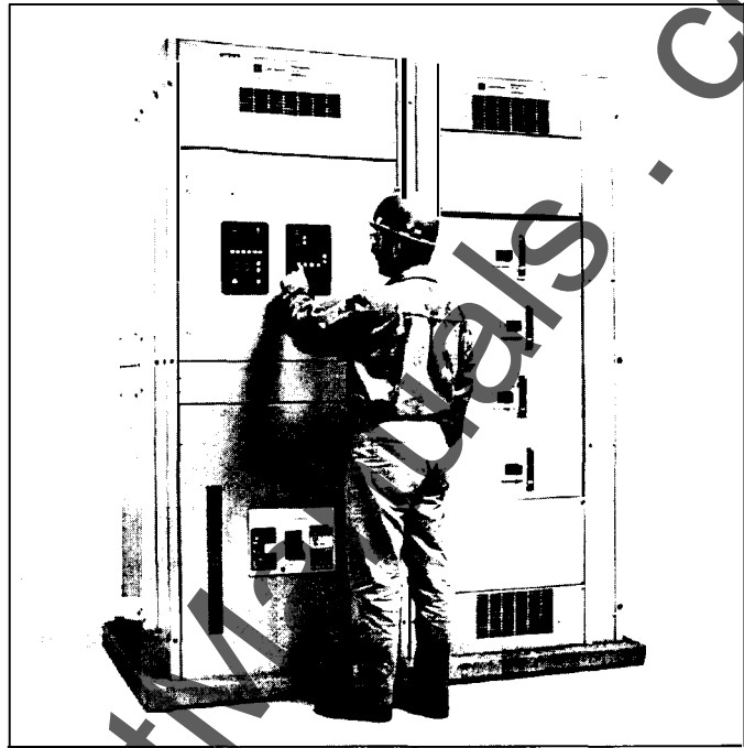
Figure 1-7 Breaker Interface Module in Service
