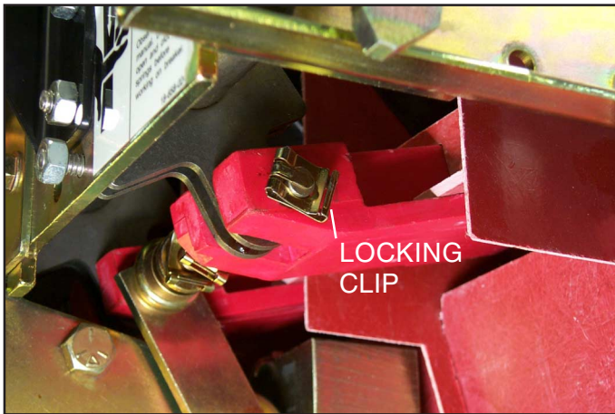
Fig. 36 Location of the Locking Clip.
