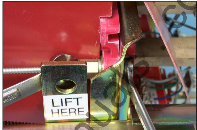
Fig. 12 Removing the Bolt from the Right Arc Chute Retaining Hardware Set.
