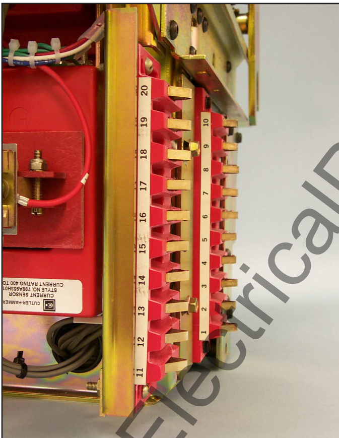
Fig. 40 Location of the Secondary Contacts.
