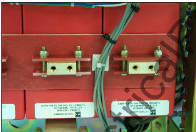
Fig. 8 Existing Breaker Wiring Secured to the Insulation Piece.
