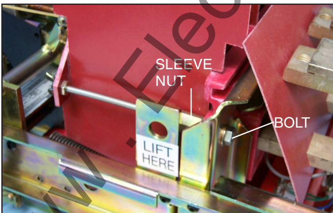
Fig. 11 Location of the Sleeve Nut and Bolt.
