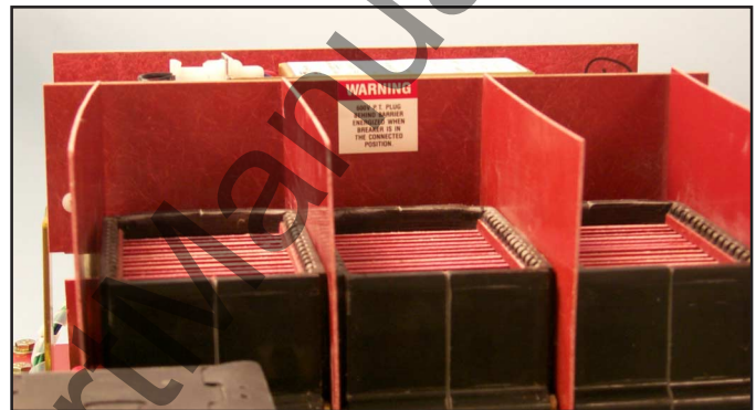
Fig. 28 PT Warning Label Installed on the Front Aux. CT Module Insulation Barrier.
