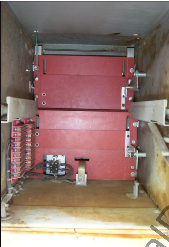
Fig. 59 The Inside of the Breaker Cell.
