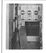
ADDED ACCESSIBILITY TO THE BUS JOINTS CAN BE OBTAINED BY REMOVAL OF REAR PLATE IN BREAKER COMPARTMENT.
