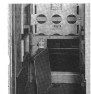
ADDED ACCESSIBILITY TO THE BUS JOINTS CAN BE OBTAINED BY REMOVAL OF REAR PLATE IN BREAKER COMPARTMENT.
